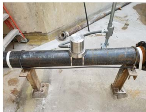
Pipe clamped properly
